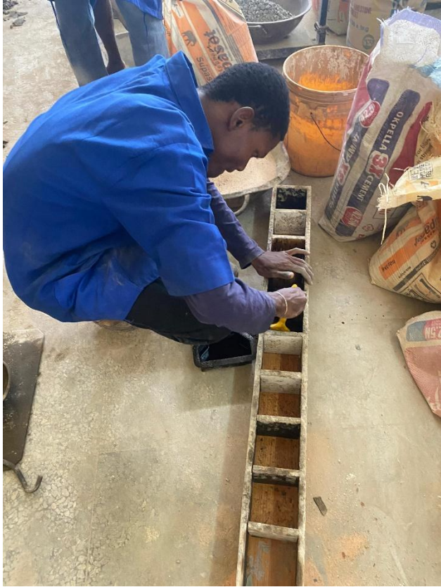
Plate 3: Casting process of concrete
