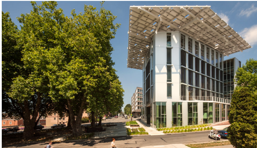
Plate 5: photo of the Bullitt center Source: bullittcenter.org
