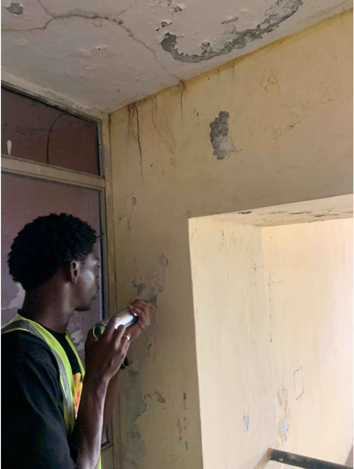
Plate 4: Schmidt Hammer Testing on Site A Ground Floor
