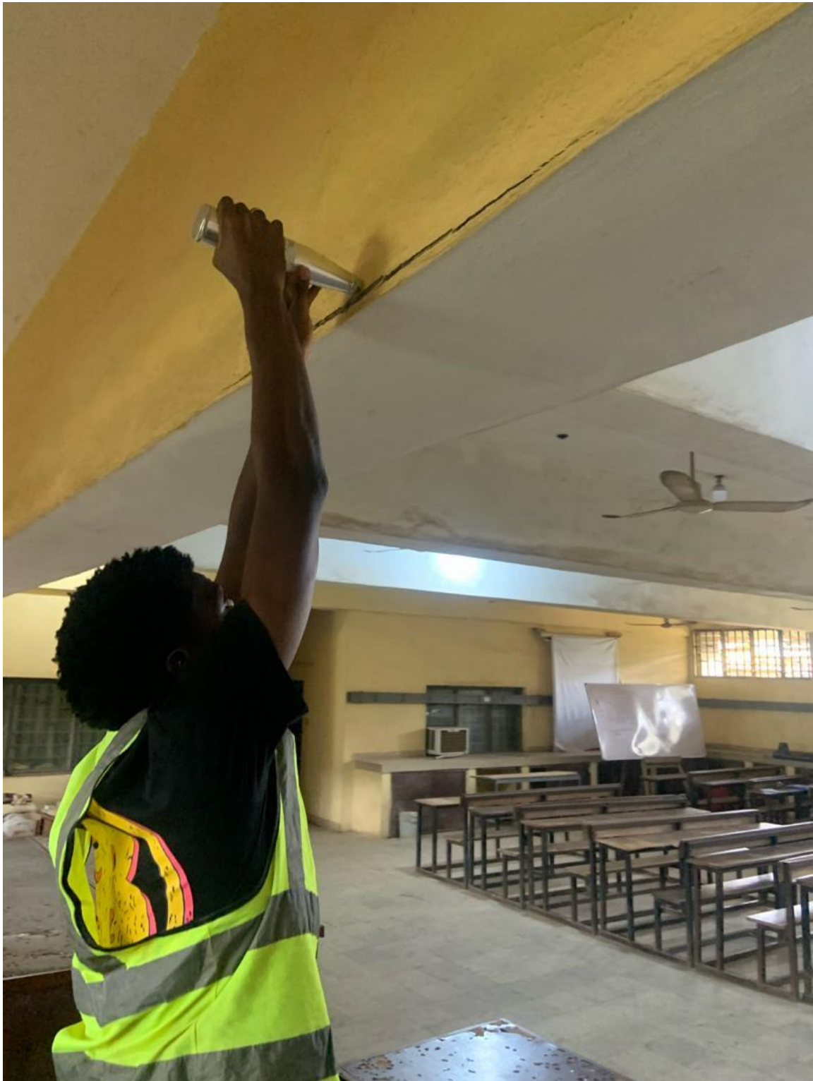
Plate 1: Schmidt Hammer Testing on Site A
