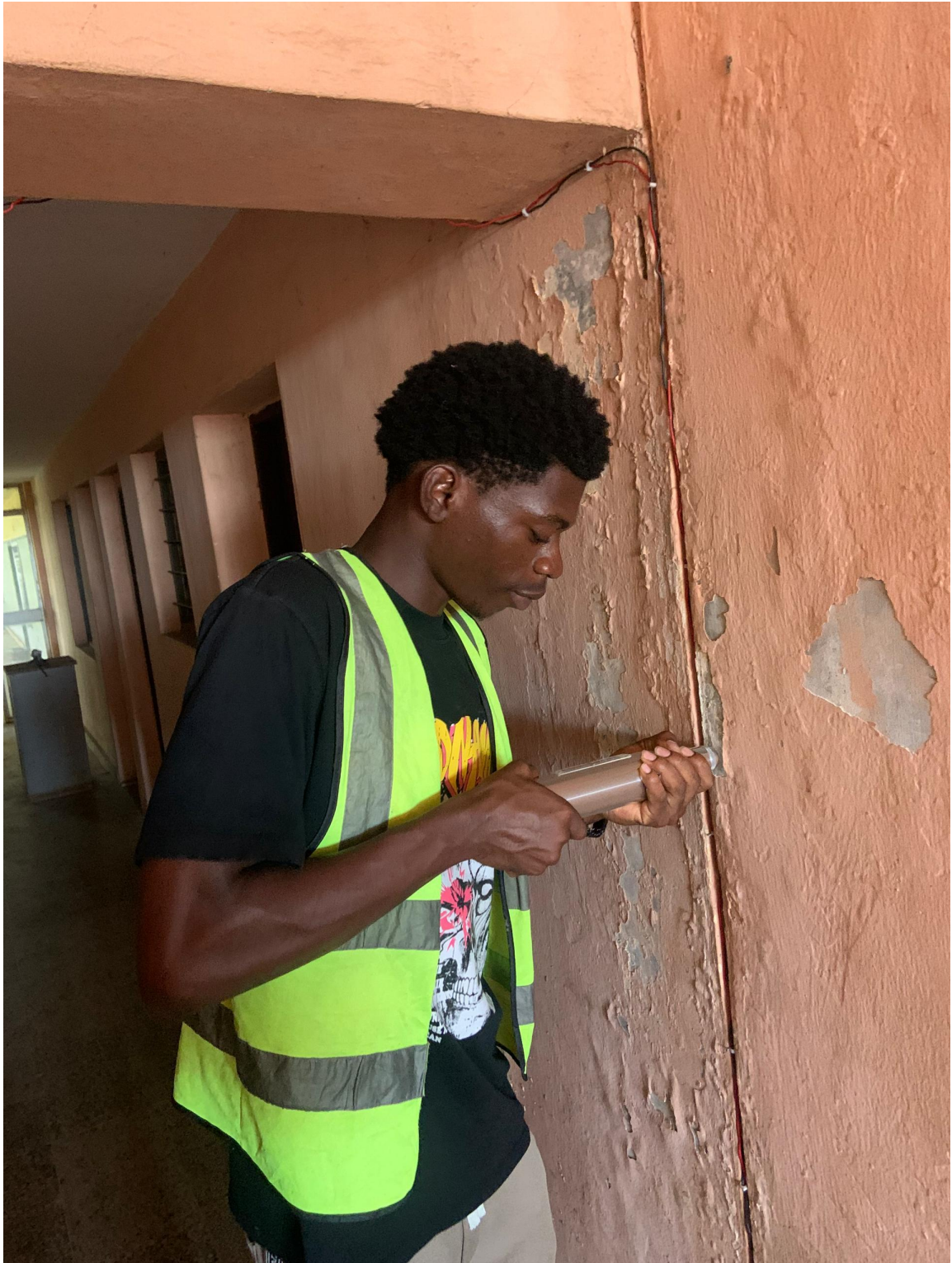
Plate 5: Schmidt Hammer Testing on Site A First Floor
