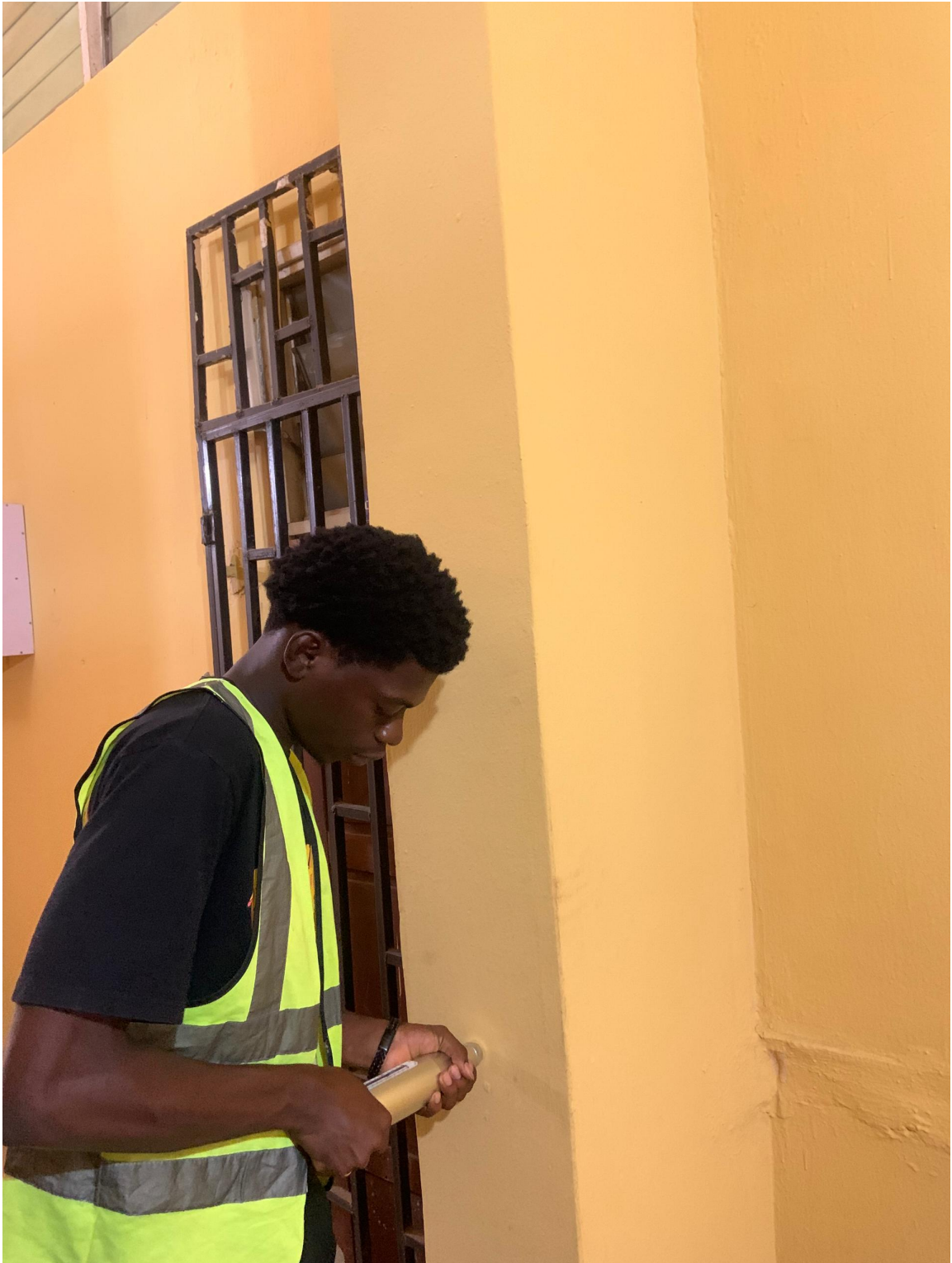
Plate 3: Schmidt Hammer Testing on Site B
