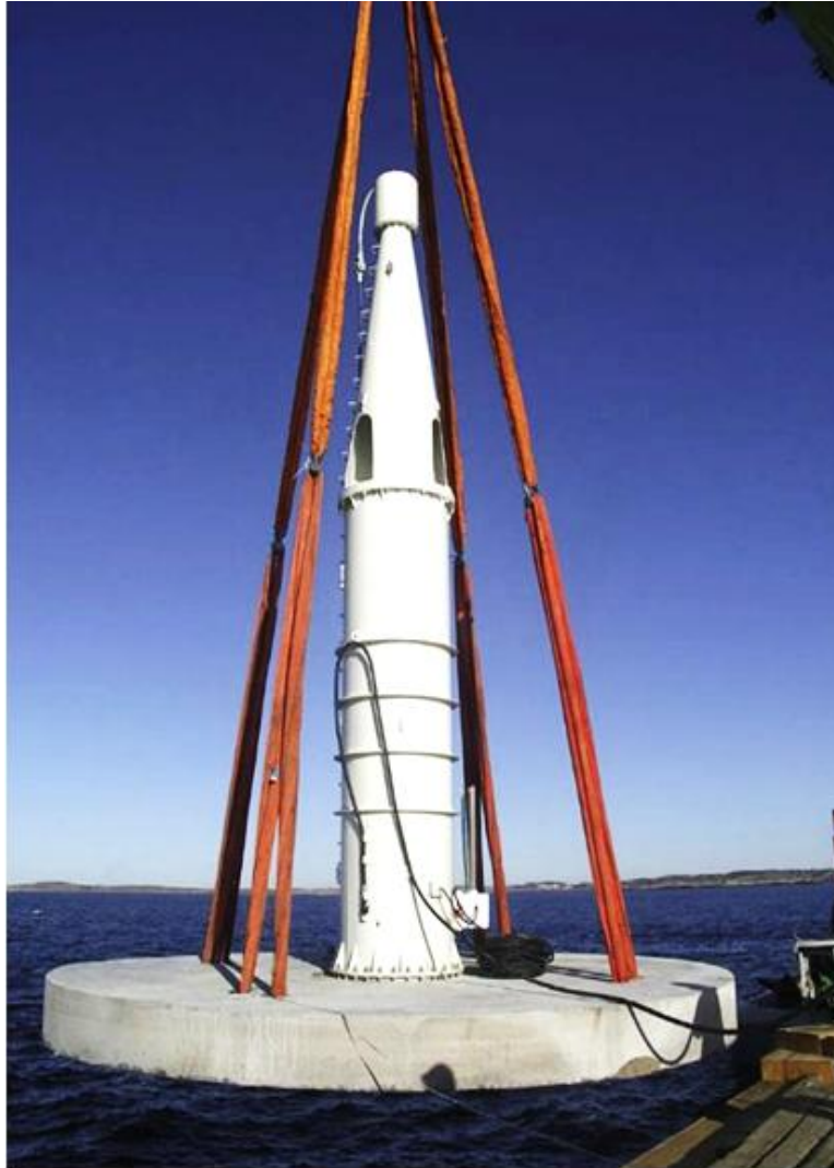
Figure 2.4: Deployment of a WEC developed by Uppsala university in the sea
