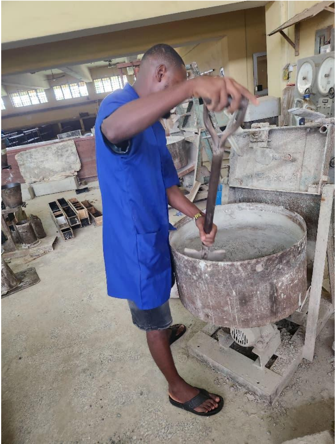
Plate C.2: Mixing of Concrete using a Concrete Mixer
