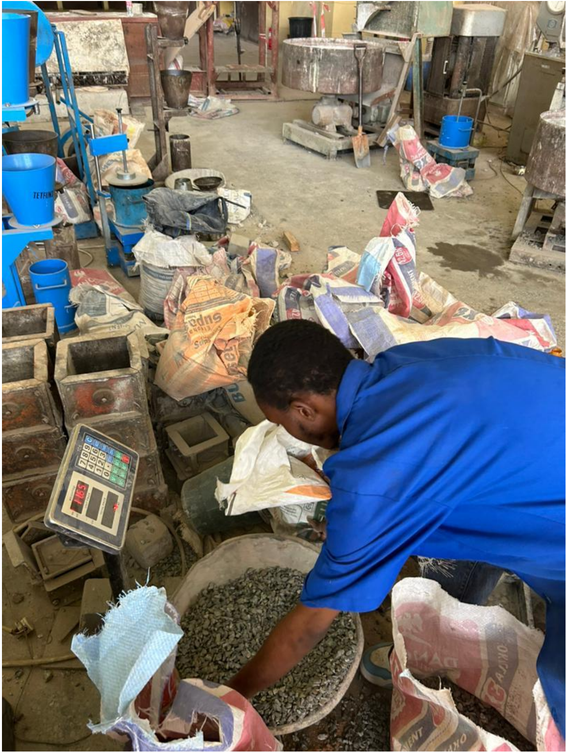
Plate 4: concrete mixing process
