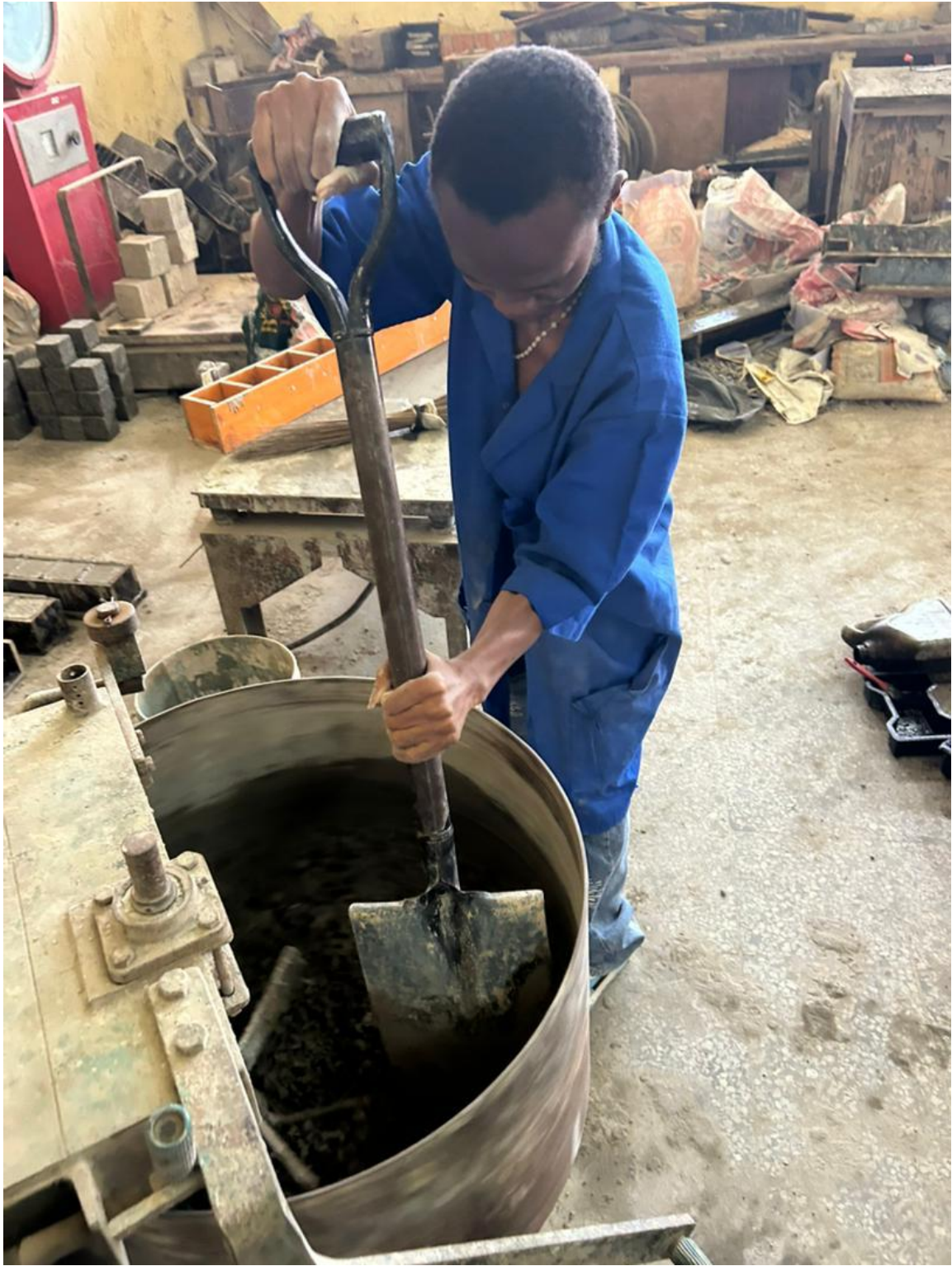
Plate 6: concrete mixing process
