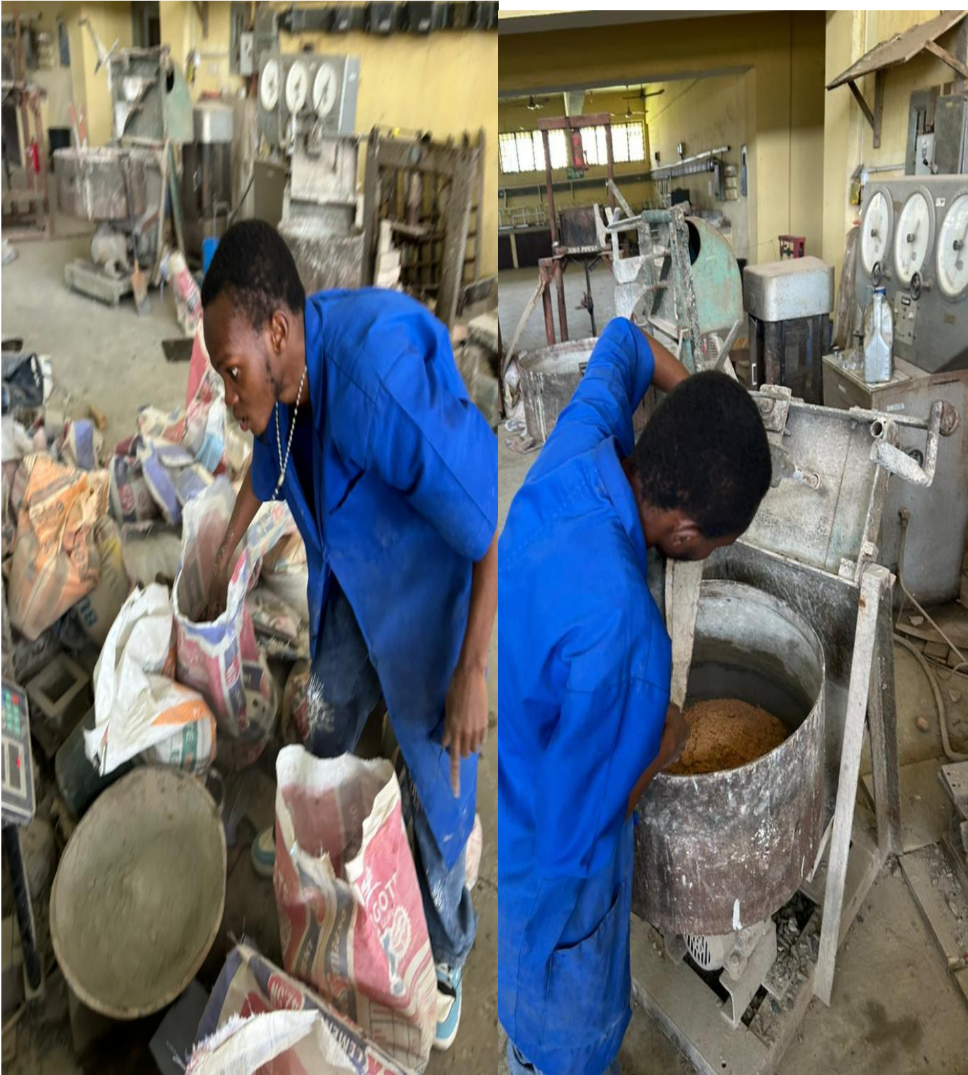
Plate 5: concrete mixing process
