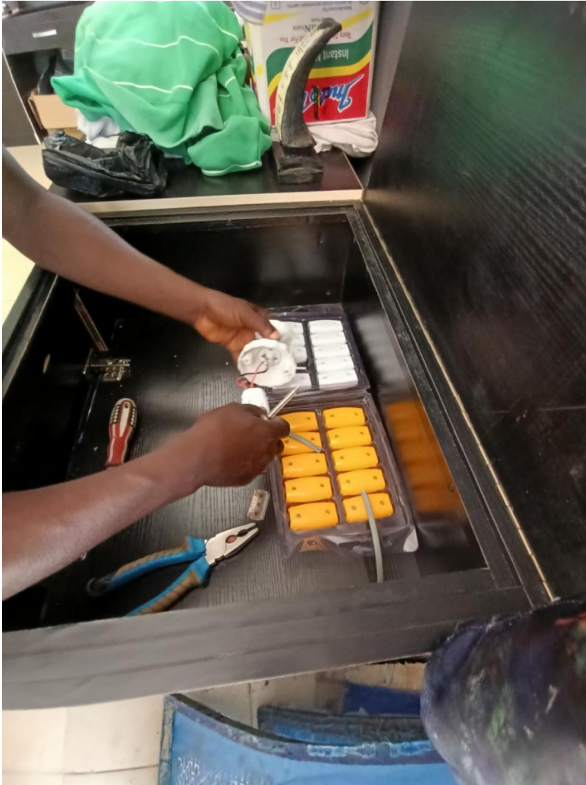
Fig.13 Fixing of light switch and lamp holder in the light boxes
