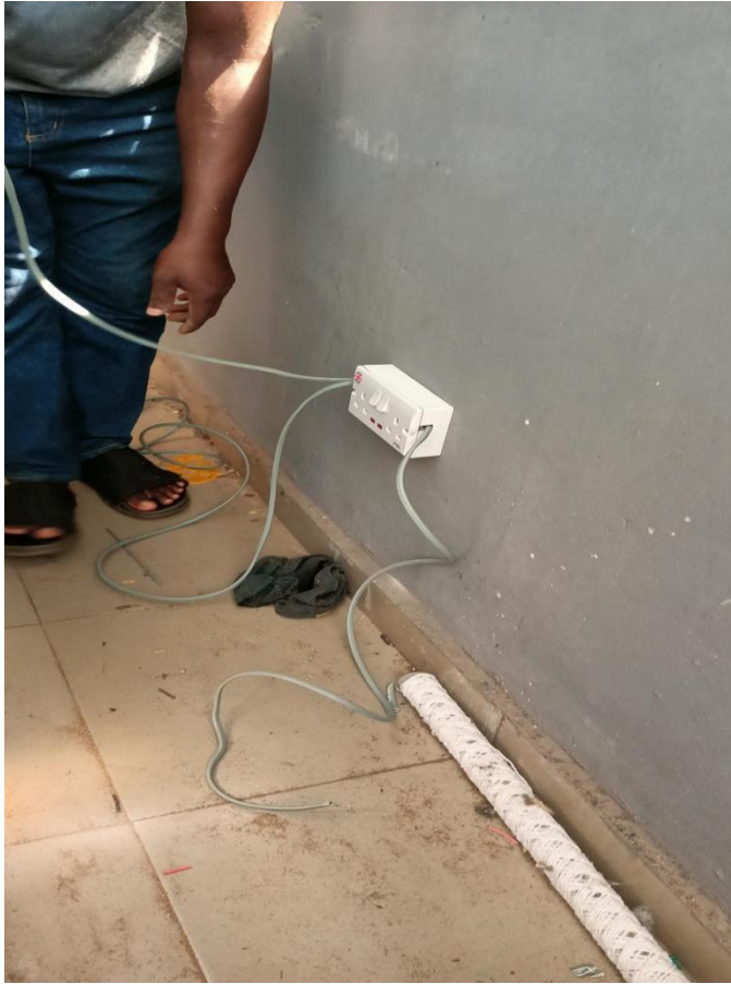
Fig.14 Fixing of electrical sockets for light boxes
