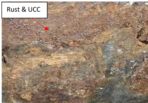
Specimen 4a (Above ground) External metal surface underneath Tape coating
