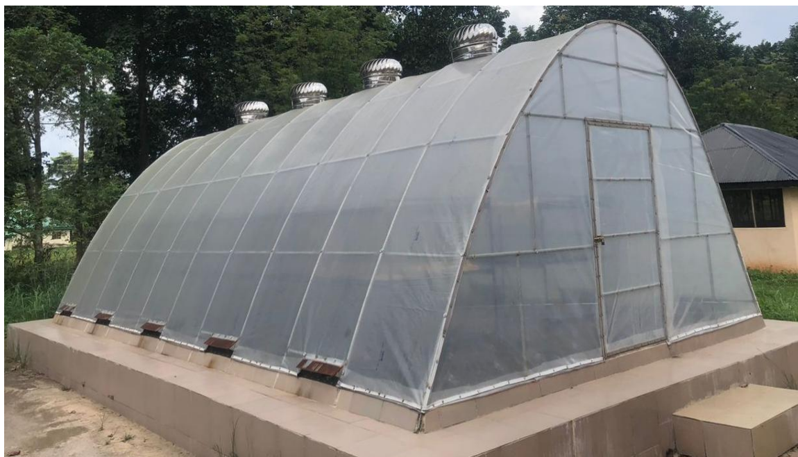
Plate 2: NSPRI Parabolic Shaped Solar Drier at the Department of Food Science and Nutrition, Faculty of Agriculture, University of Benin (UNIBEN).
