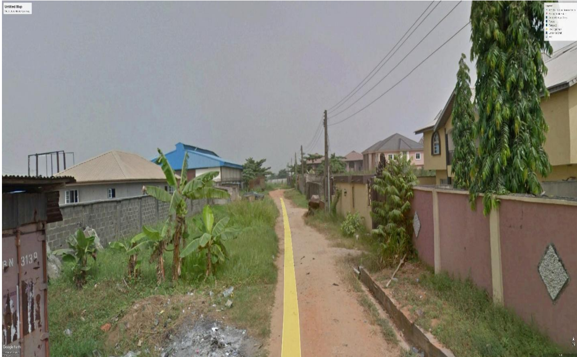
Fig:4.4.3: Street condition in Amuwo-Odofin estate showing signs of decay and abandonment.
