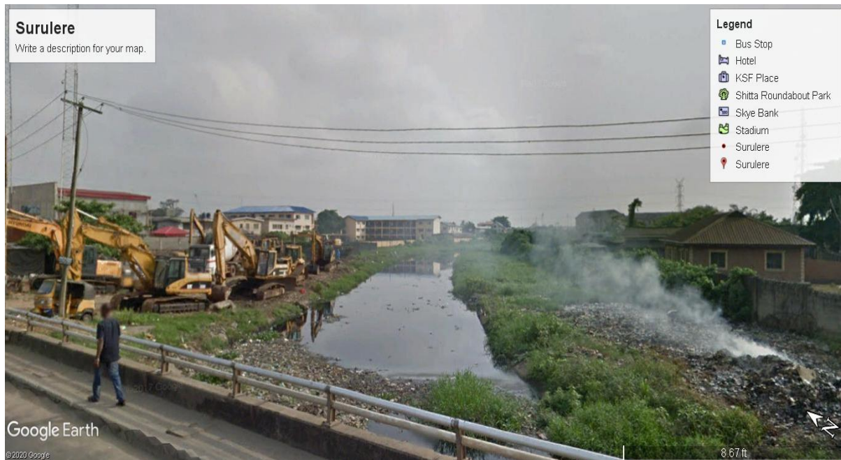
Fig. 4.7.4: Flooded Drainage filled with waste materials in Surulere.
