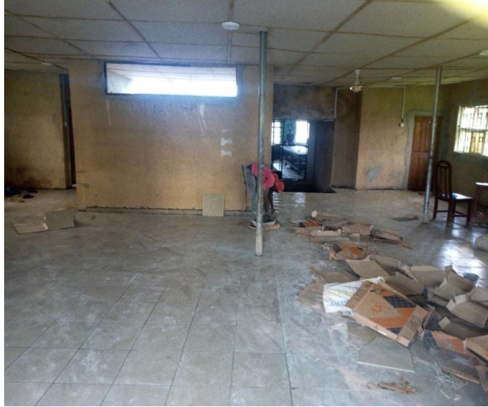
Fig. 4b: Fixing of the Tiles Photo Credit: Adaimoni Raymond
