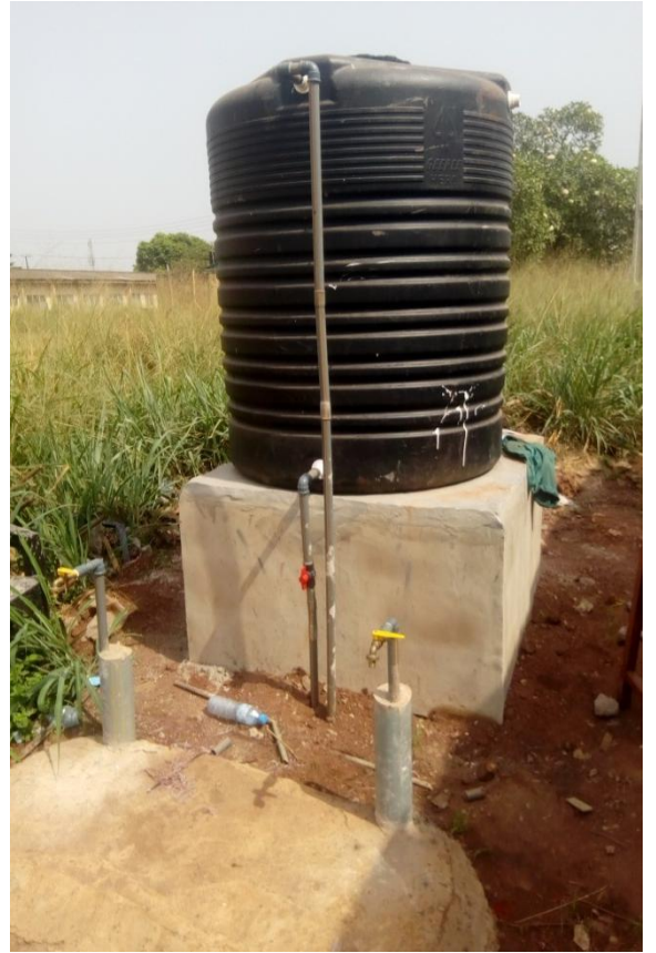
Fig. 10b: Finished Borehole and Taps Photo Credit: Oyedele Joshua
