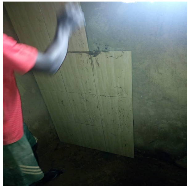
Fig. 4a: Fixing of Tiles Photo Credit: David Eniye
