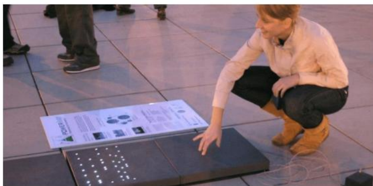
Figure 2.5. POWERleap tiles installation (Redmond, 2021).
