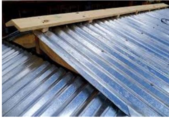
FIGURE 2.11 CORRUGATED IRON SHEETS
