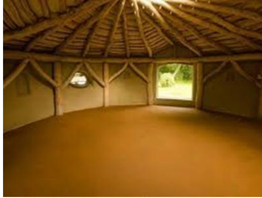
FIGURE 2.12 EARTH AND CLAY FLOORS
