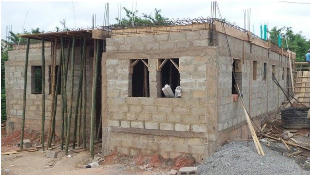
FIGURE 1.2 HOUSE UNDER CONSTRUCTION
