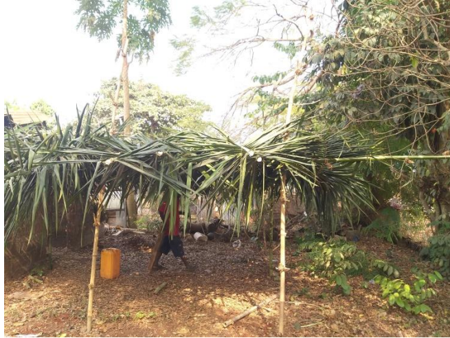
Plate 3.1: Construction of the insectarium with locally sourced materials
