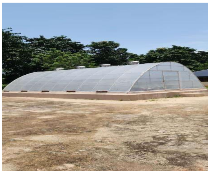
Figure 4.32: Modern solar dryer facility observed during fieldwork in Oredo LGA, used for hygienic and efficient preservation of vegetables and fruits.
