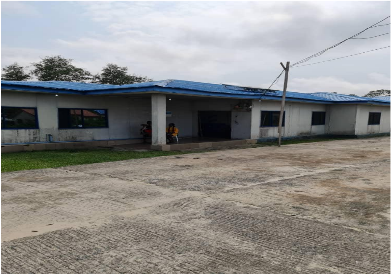
Pix. 1: Front view of Ugborodo Health Centre, Ode Ugborodo Town, Warri South-West Local Government Area, Delta State, Nigeria.
