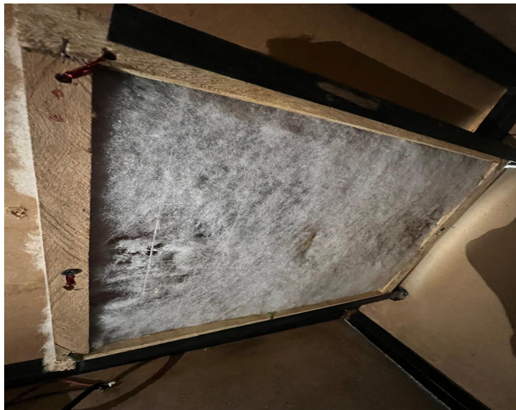
Figure 3.6 Wood insulated for extractor hood
