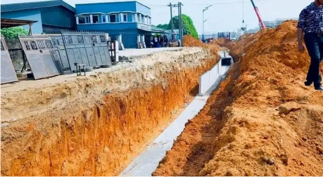
Figure 1: Drainage under construction.
