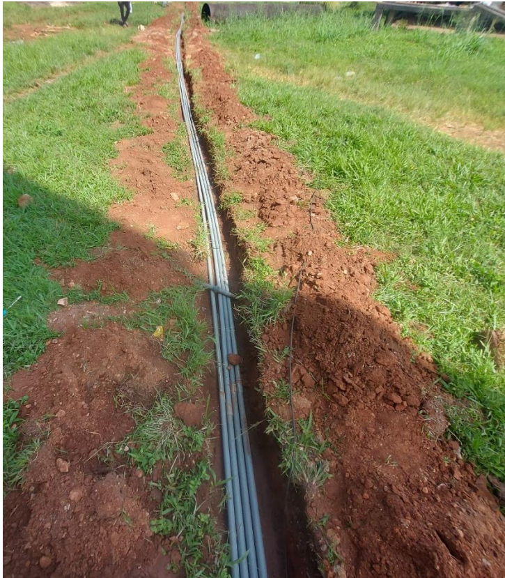
Figure 23 - pictures of the pipe laying process
