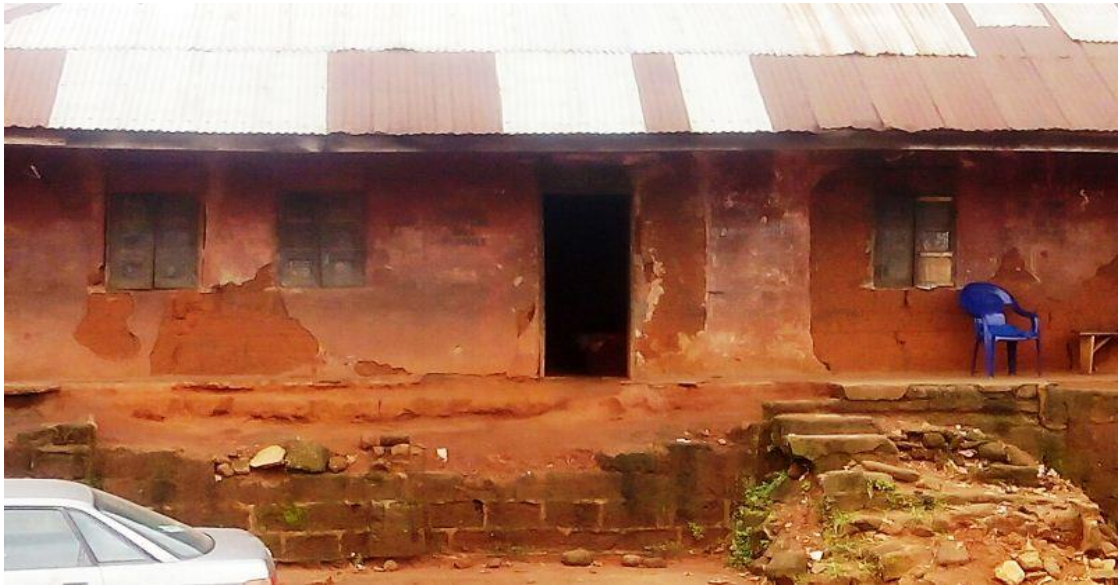
Plate 4. 1: Mud wall bungalow found in zone C1 off ring road. (Poor quality house) Source: Researcher's field work, 2016
