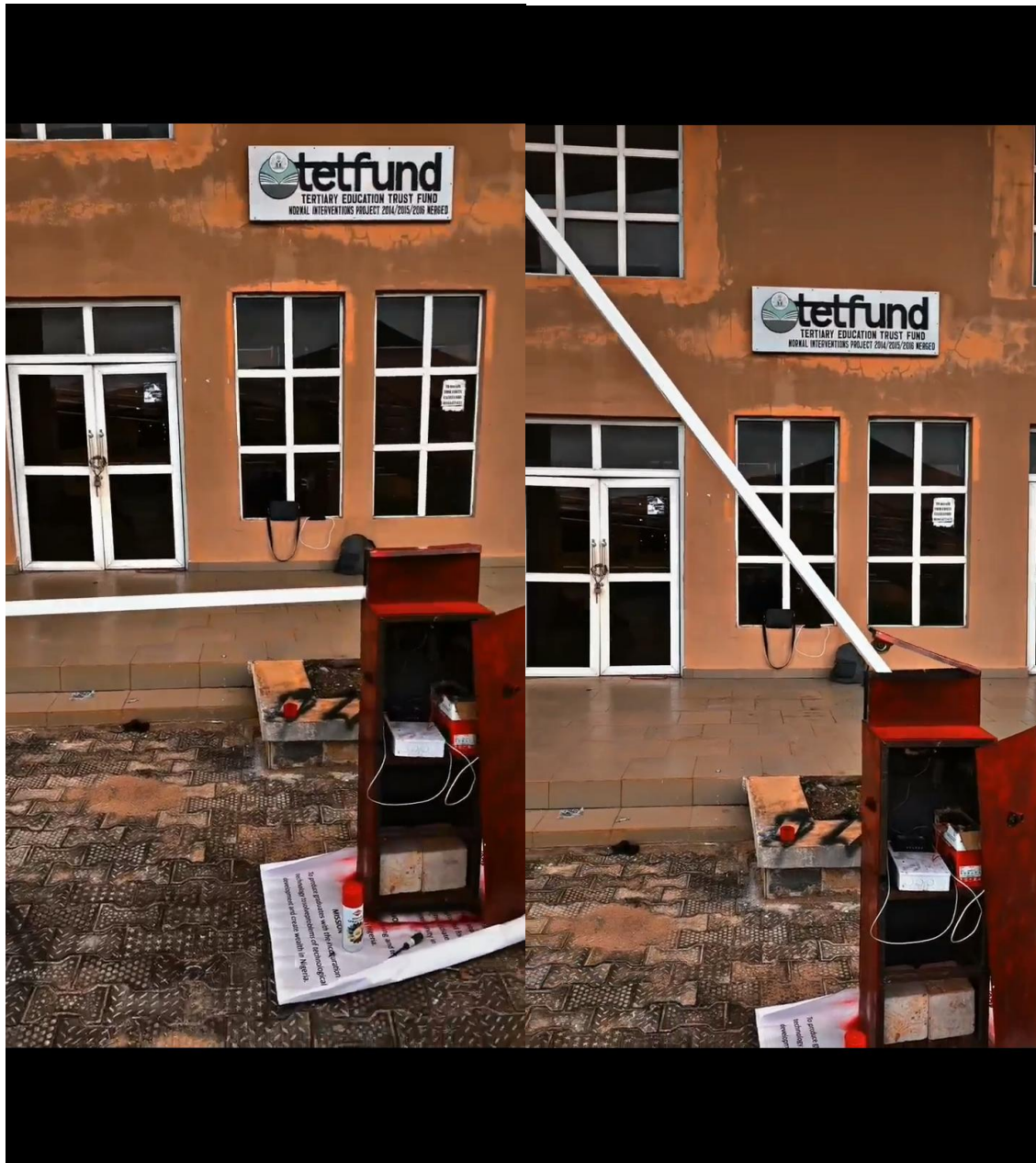
Fig 3.15 System Undergoing Testing
