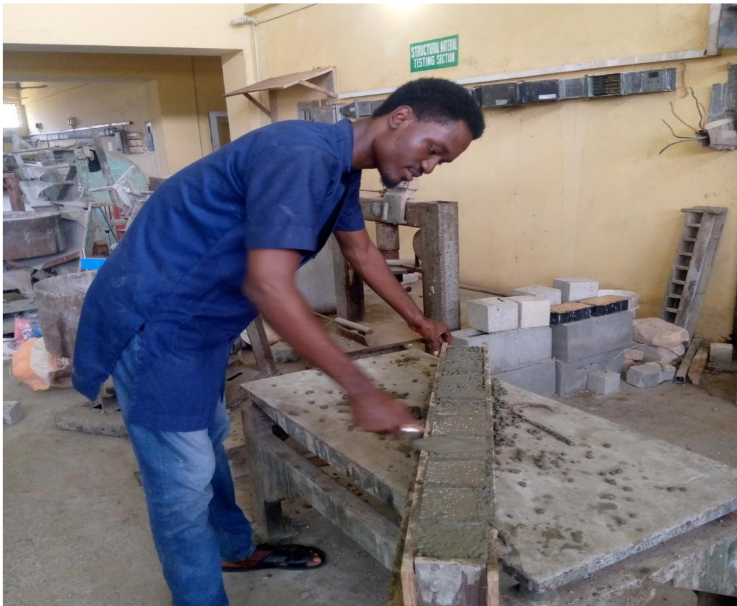
Figure A - 5: Student levelling the surface of a compacted fresh concrete
