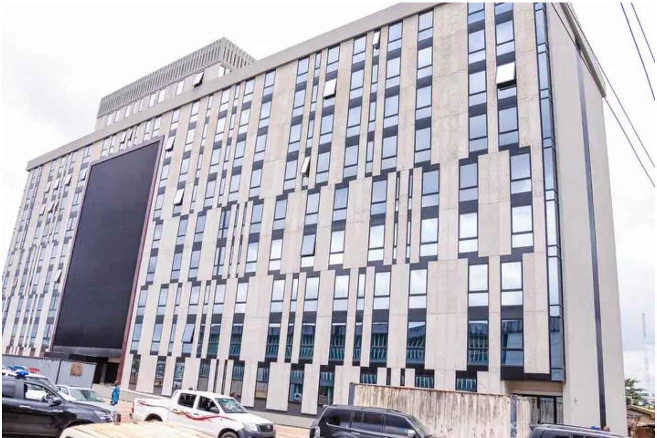
figure 4.4: A view of on-going renovation of office Block B, 90% completion.
