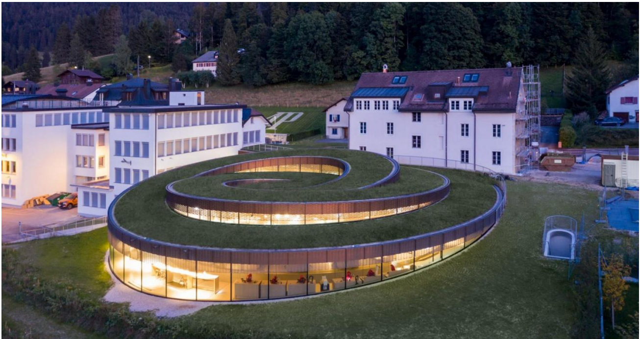
Figure 4.6: Aerial view of the Musée Atelier Audemars Piguet (Source: Iwan Baan, retrieved from Arch daily 2022)
