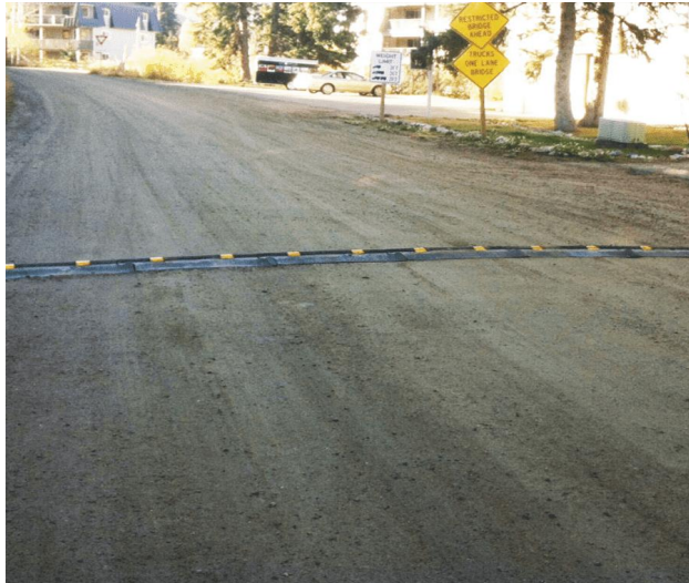
FIGURE 2. 15 GRAVEL ROAD SPEED BUMP (SOURCE: RUBBERFORM, 2023)
