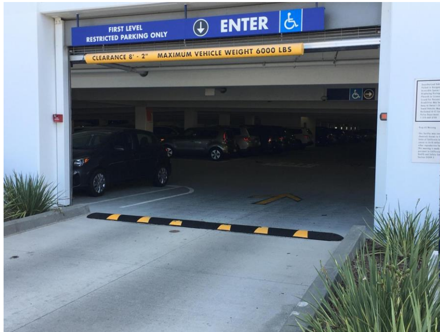
FIGURE 2. 18 PARKING LOT SPEED BUMP (SOURCE: CAMINO, 2023)
