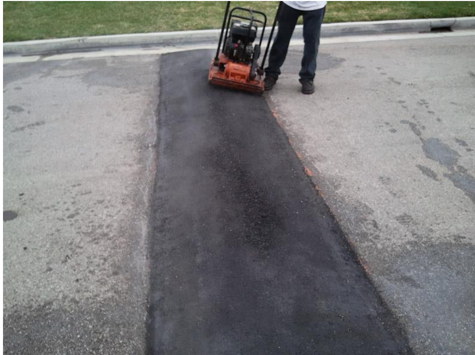
FIGURE 2. 21 ASPHALT SPEED BUMP (SOURCE, EMPIRE, 2023)
