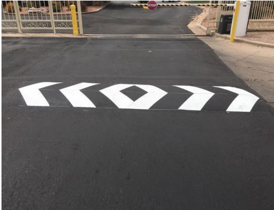
FIGURE 2. 14 DRIVEWAY SPEED BUMP (SOURCE: SWAINE, 2023)
