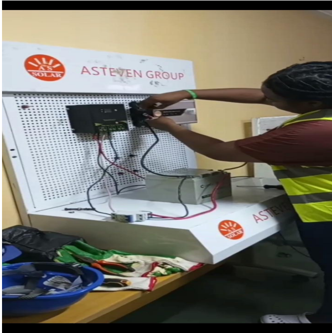
Sourced from field work showing how the connection of Inverters, charge controllers and battery
