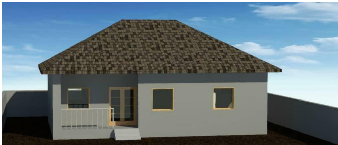
Plate B-2: Building before collapse
