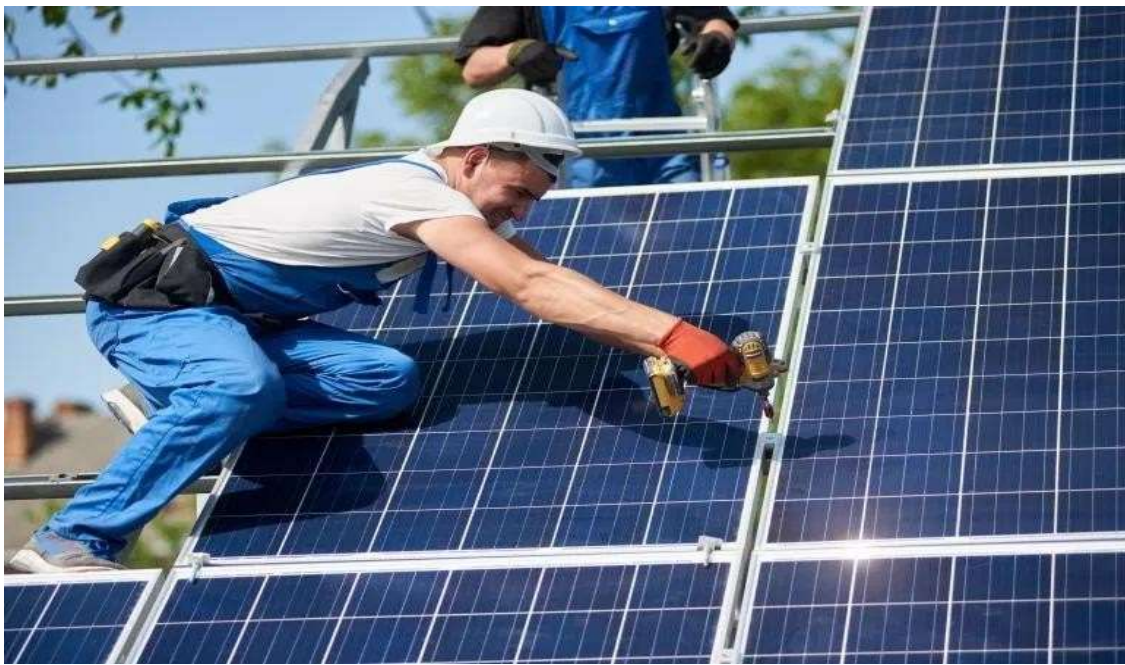
Figure 2.3: Professional technician installing solar panel to metal platform using screwdriver (Benjamin, 2019).
