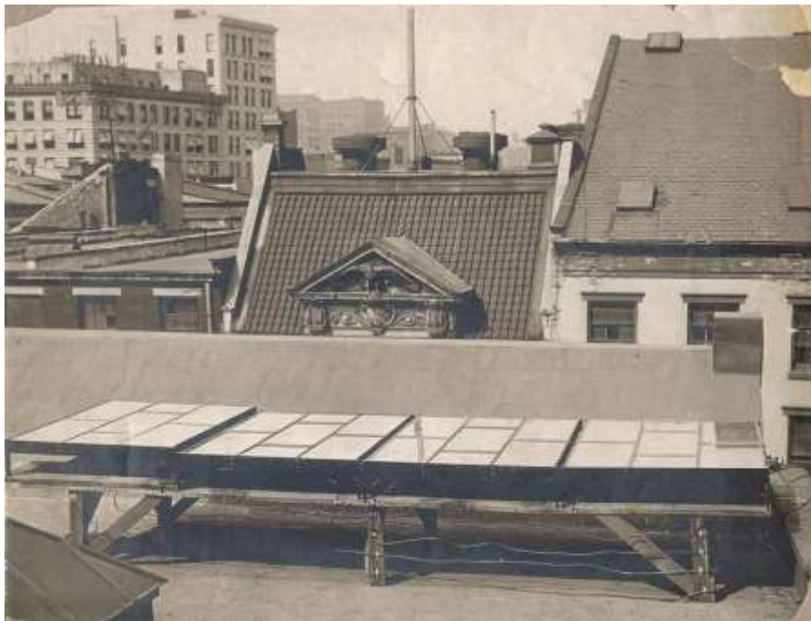
Figure 2.1: Charles Fritts installed the first solar panels on New York City rooftop in 1884 (Elizabeth & D.Lawrence, 2019)
