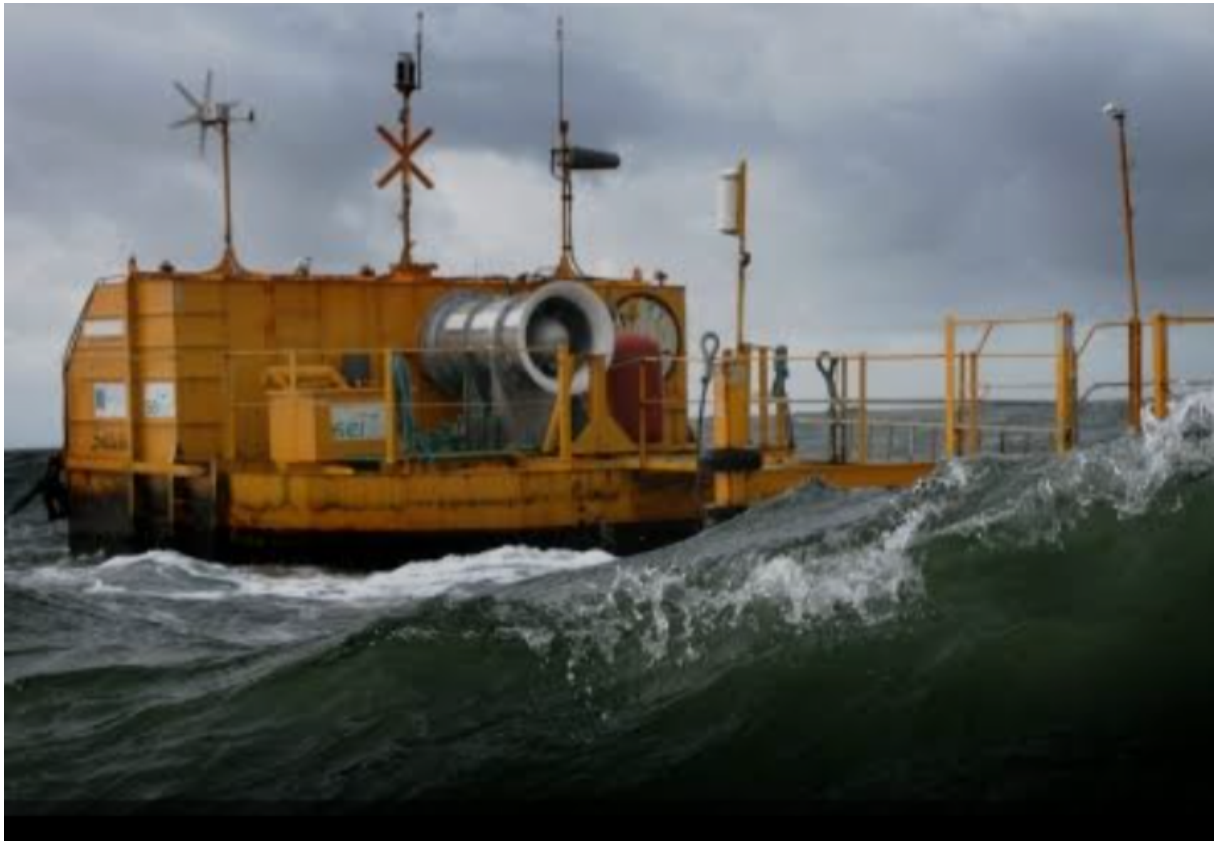
Figure 2.11 Oscillating water column installed in Australia
