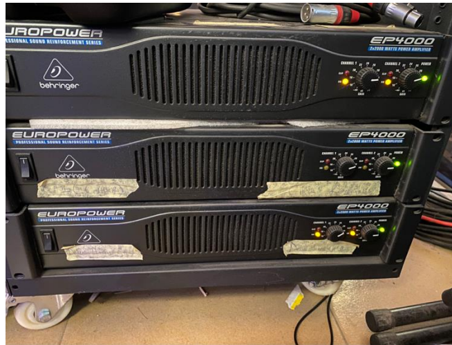
Figure 2.2: The Behringer EP4000 audio power amplifiers in a rack cabinet.
