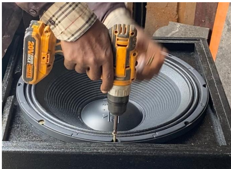
Figure 3.12: the transducer being held into place by screws.
