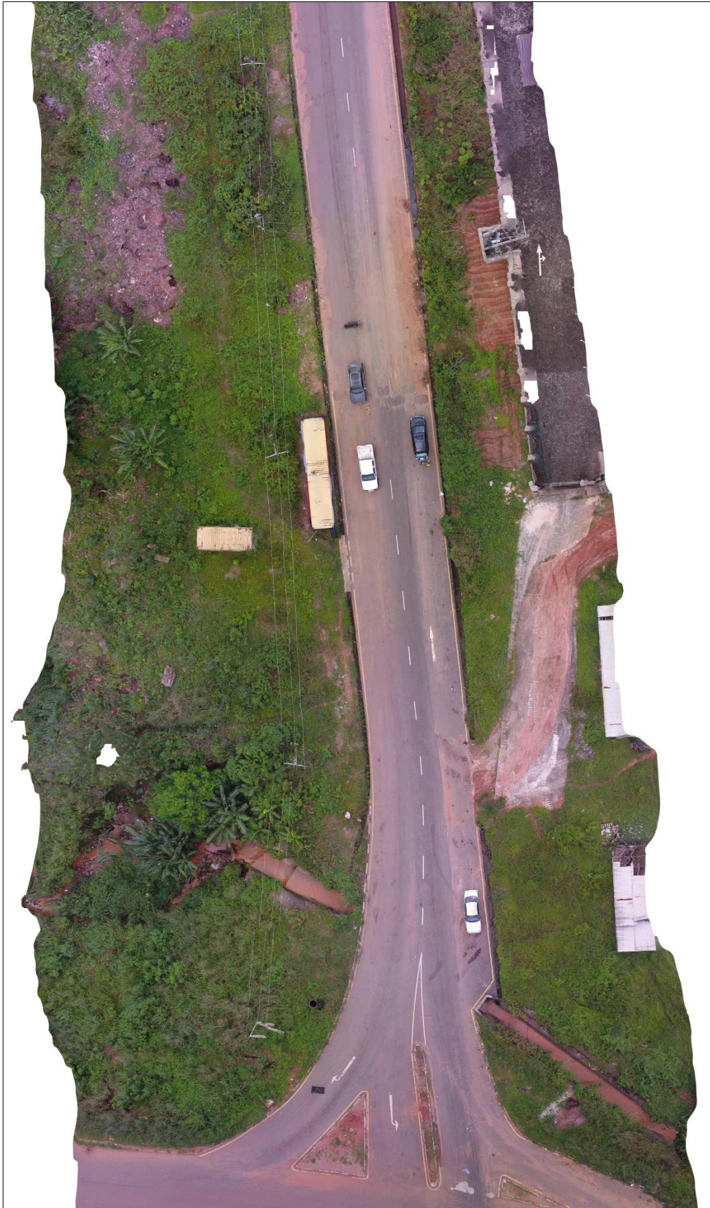
Figure 4.2g: Aerial view showing beginning of Temboga road captured using Phantom 4 Pro
