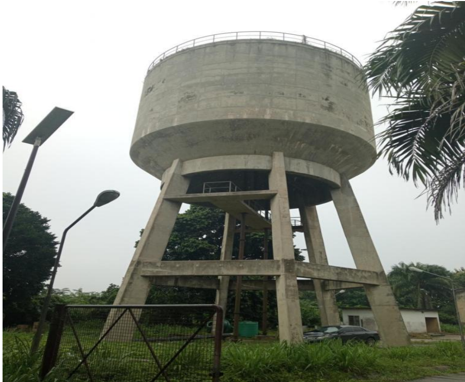
Figure 3.4: Concrete Overhead Tank at the Uniben Water Scheme
