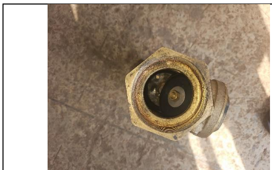
Figure 3.11: Check Valve
