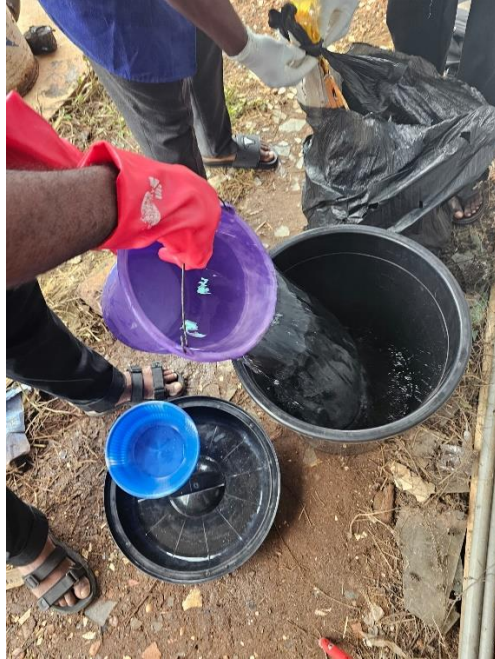
Figure 4.11: Addition of Water into Mixing Container
