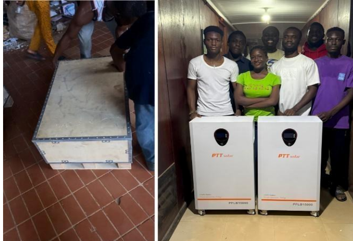
Figure 4.5 Unboxing and Inspection of Batteries
