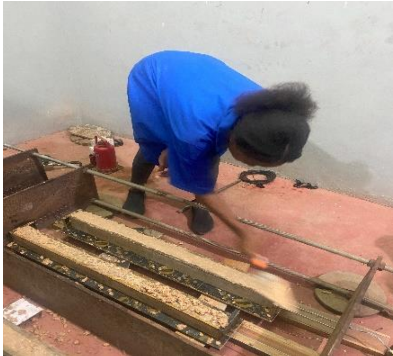
Figure 3.4: Casting of concrete beam and cubes
