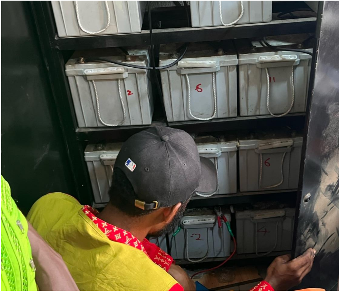
Figure 4.3: Installation of Battery Bank
