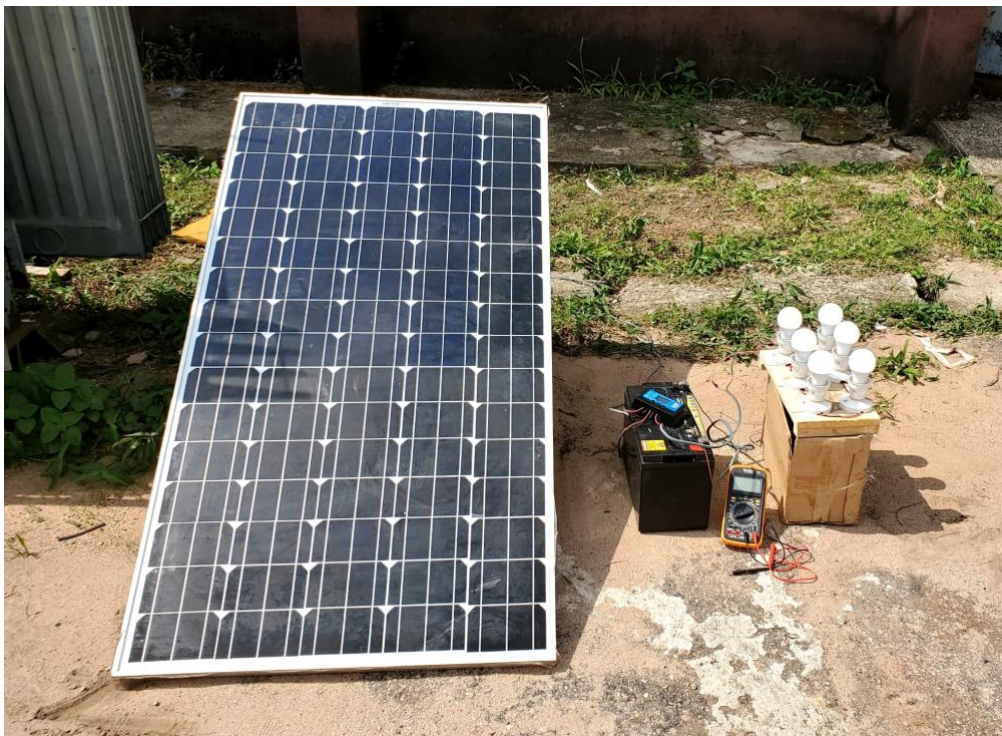
Figure 3.9: Physical Implementation of the PV system
