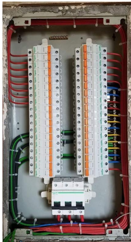
Figure 4.5: Distribution Board
