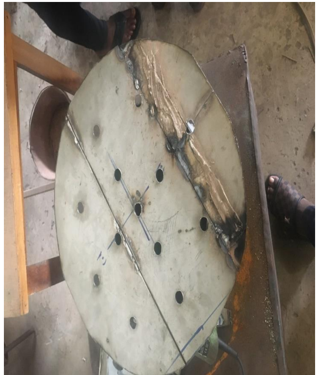
Holes drilled on the Rotating Plate for the Rubber Fingers
