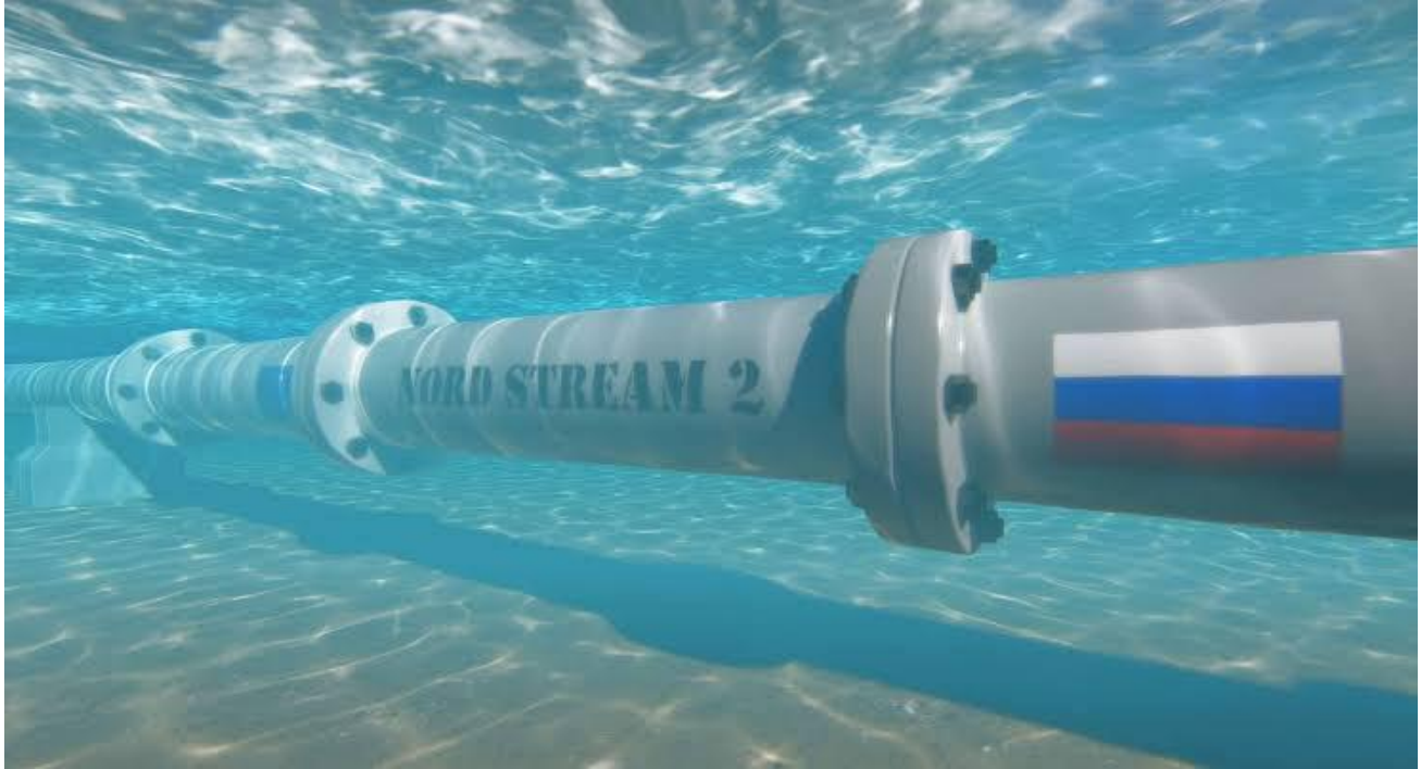
Fig 1.4.2 Nord Stream 2 gas pipeline Source:(OE Digital, 2023)
