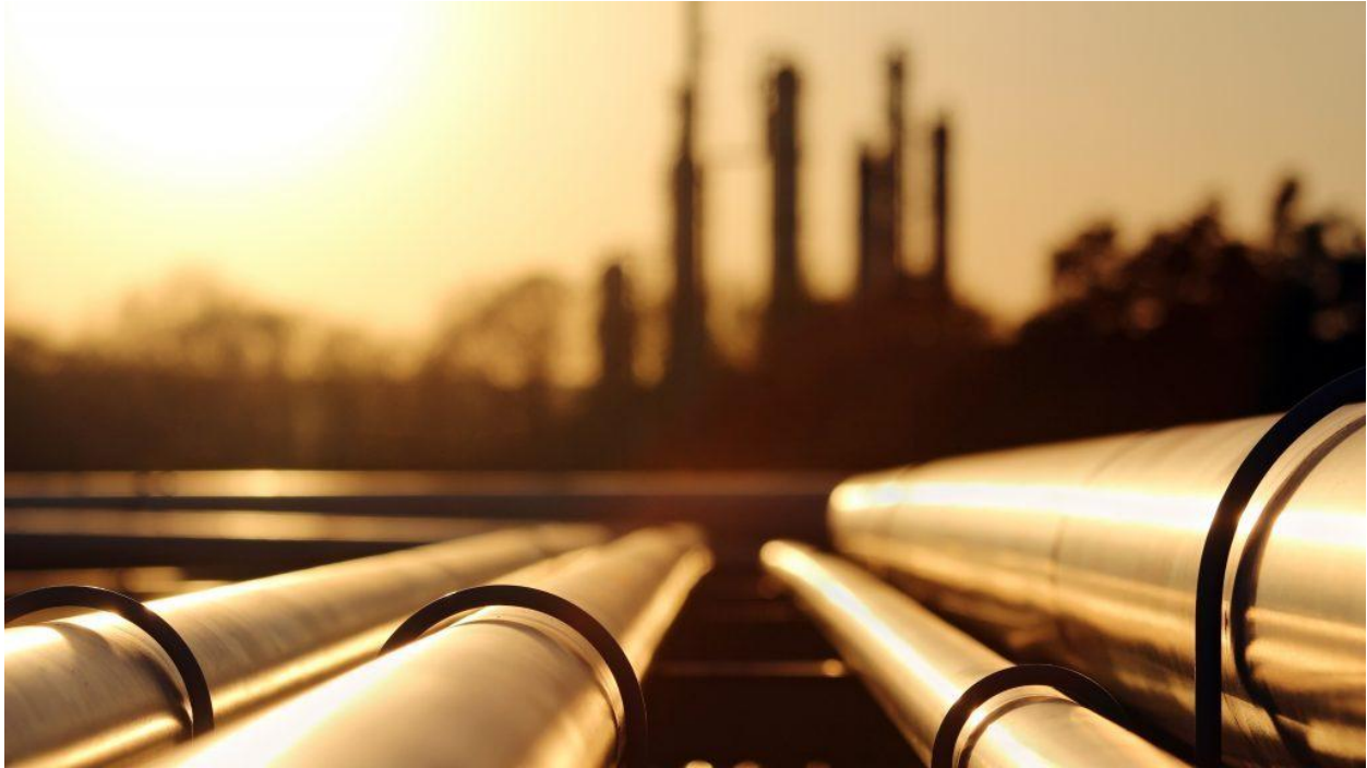
Fig 1.4.5 West-East Pipeline Source: (constructconnect, 2025.)
