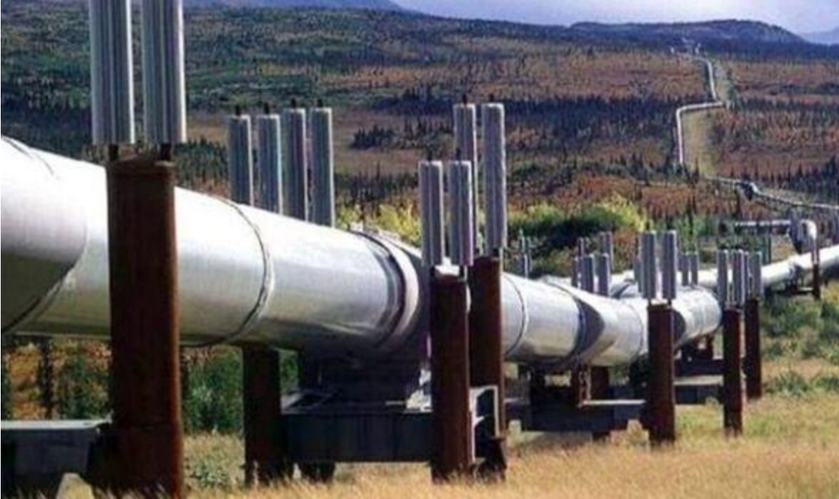
Fig 1.4.4 Keystone Pipeline Source: (Express.co, 2025.)
