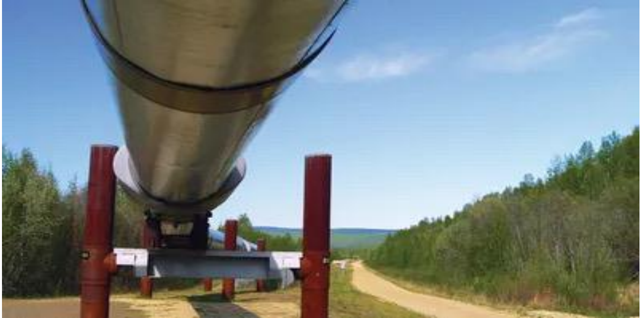
Fig 1.4.1: Ground-level view of an elevated portion of the Trans-Alaska Pipeline, Alaska, U.S. Source: (Encyclopaedia Britannica, 2023.)
