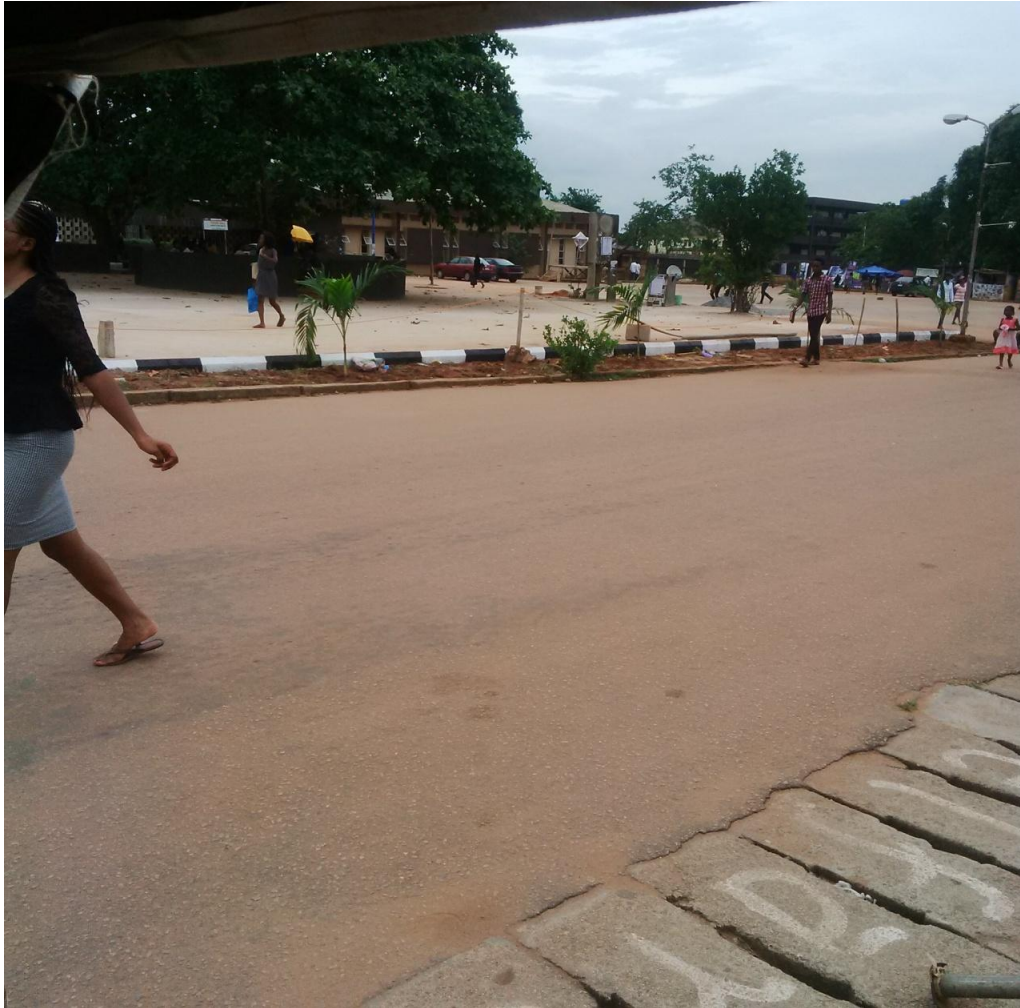
Plate 4.13: Hall Two Car Park
