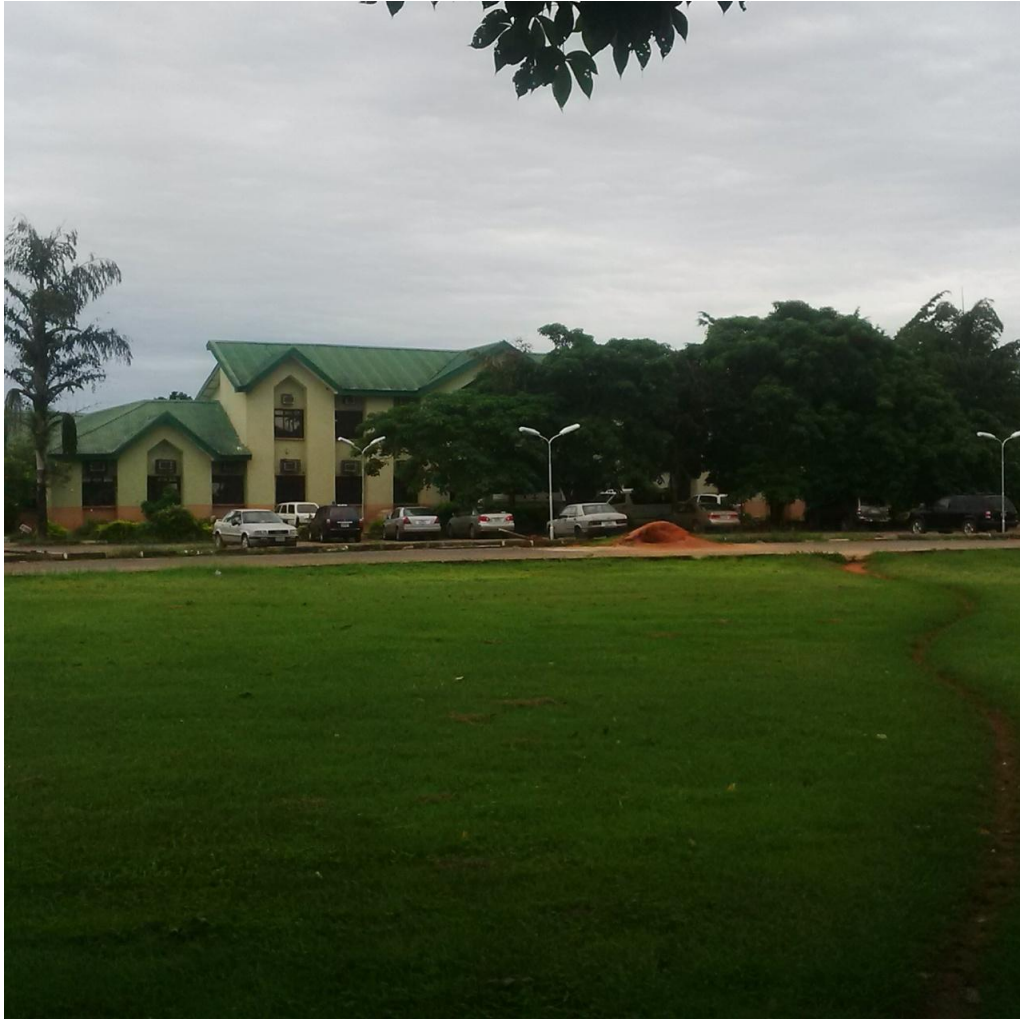
Plate 4.3: Health Centre Car Park
