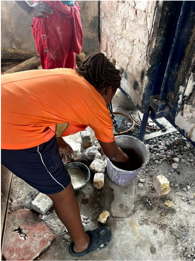
FIGURE 8 Preparation of the mortar. Photograph by Nnamani Felix.
