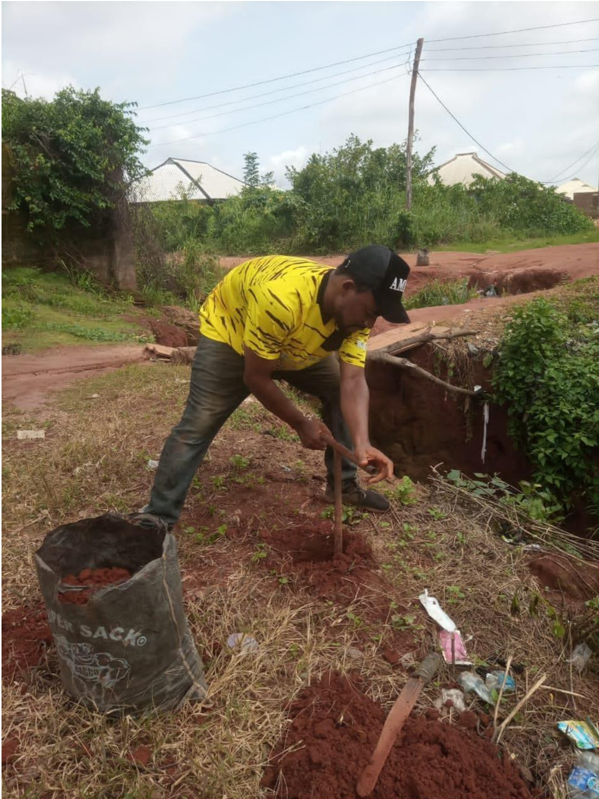
COLLECTION OF SOIL SAMPLE FROM SITE
