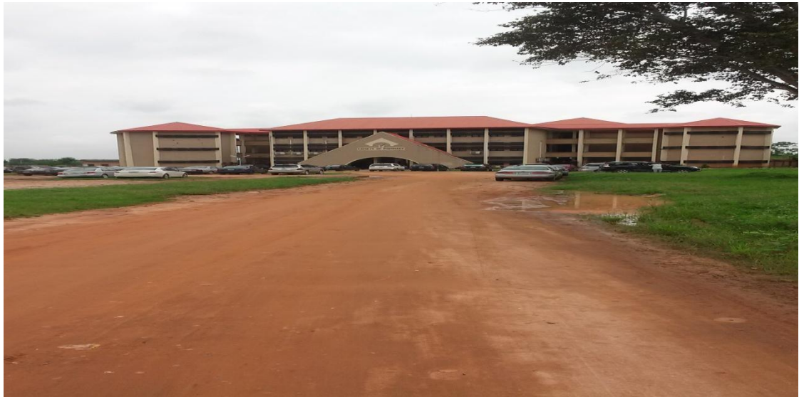
Plate 4.23: new pharmacy building
