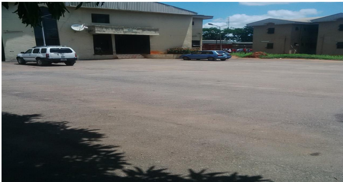
Plate 4.11: Hall Five Car Park
