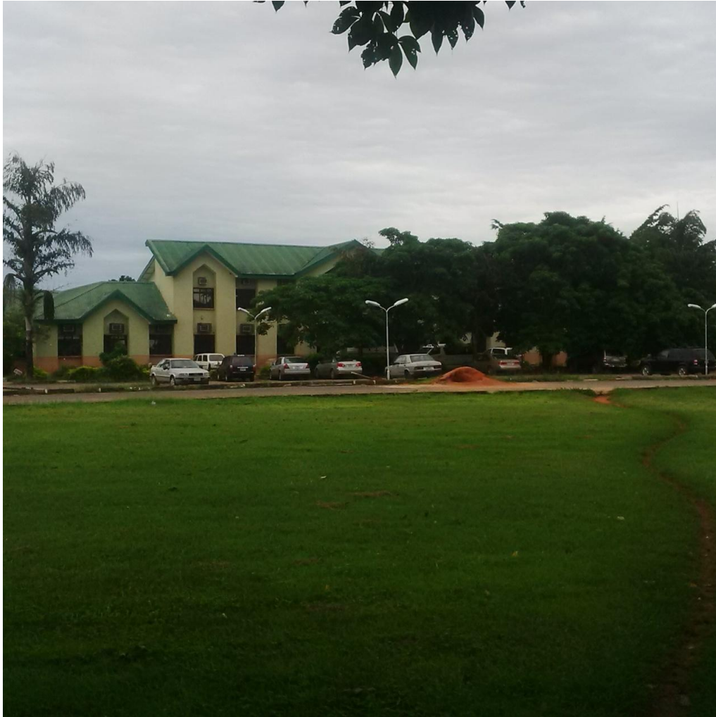
Plate 4.3: Health Centre Car Park
