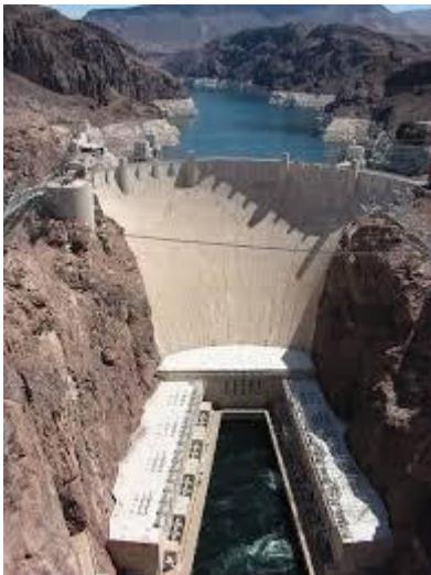
Fig. 2.1: Hoover dam which is the largest dam in the world
